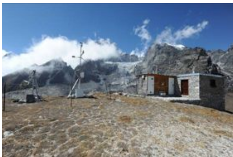
Figure 3. The NCOP Observatory in 2006: the door on the right provides access the battery room, while the left part houses the instrumentation. Through the aluminium roof, four sampling lines allow the sampling of gas and aerosol particles. A live webcam imager is also visible, allowing the real-time image available on the website http://evk2.isac.cnr.it/
